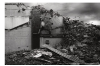
B0017094 Wall and Slope of Silo 5 7 000 kr Upplaga 15
